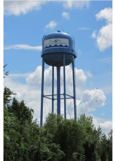
New Hwy. 97 Elevated Tank (2016)
