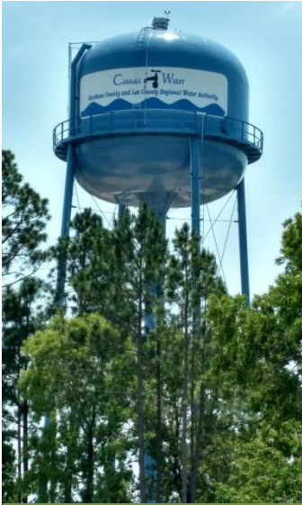
New Red Hill Elevated Tank (2017)
